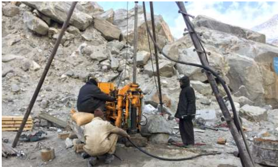
Photo 4-2 Drilling Rig at BH-02 Sediment Flushing Channel .
