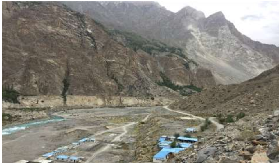
Photo 6-6 Proposed Alignment of Penstock.
