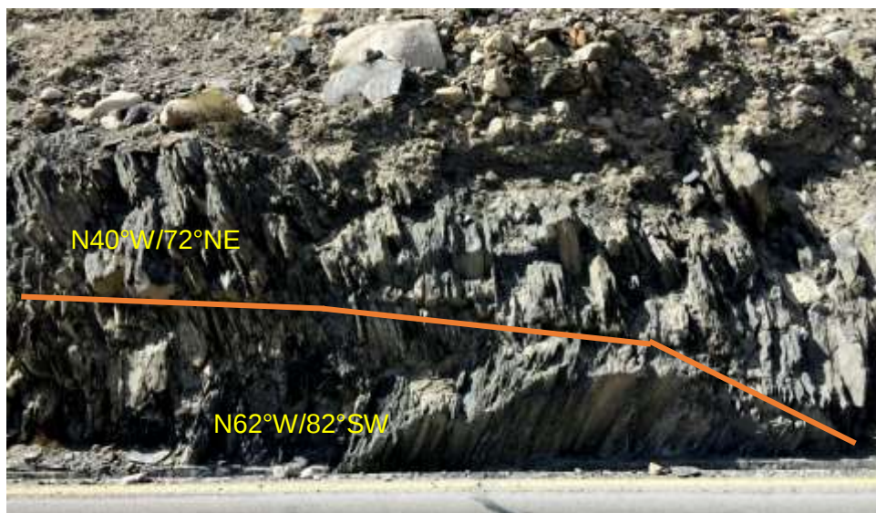
Photo 8-8 Change of Dip along Shear joint.
