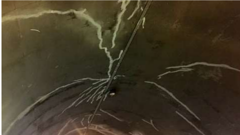
Photo 8-15 View of Recently Generated Joints Tunnel-2.
