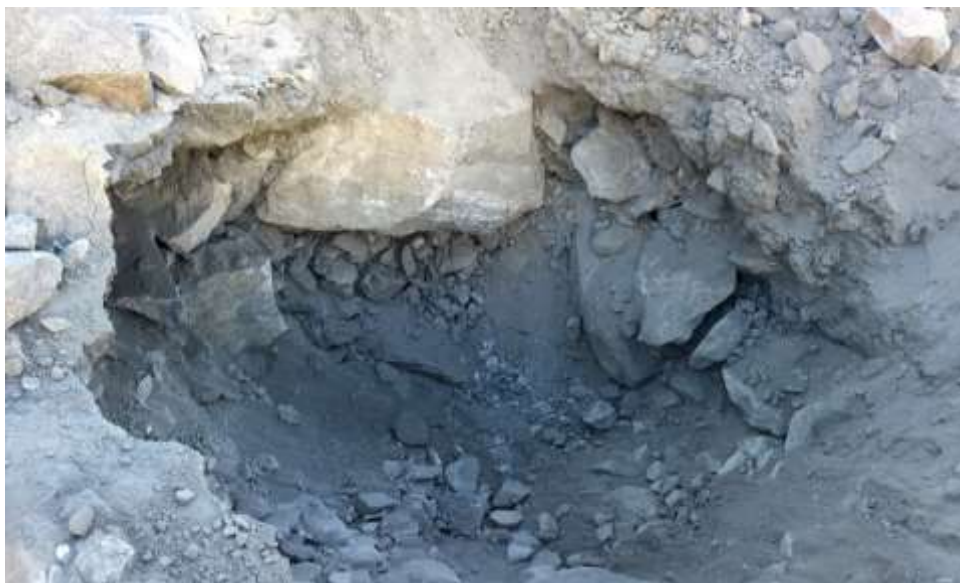
Photo 7-6 View of Slided Mass in TP-6 at Left Side Slope of Hunza River.
