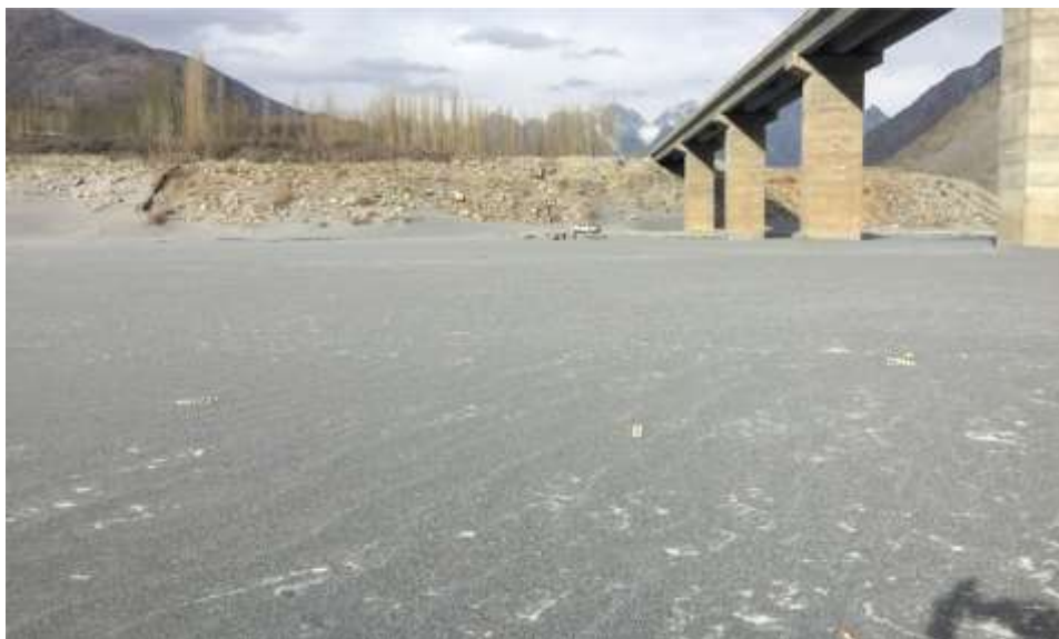
Photo 7-1 Quarry Area Selected for Sand near Shishkat Bridge.
