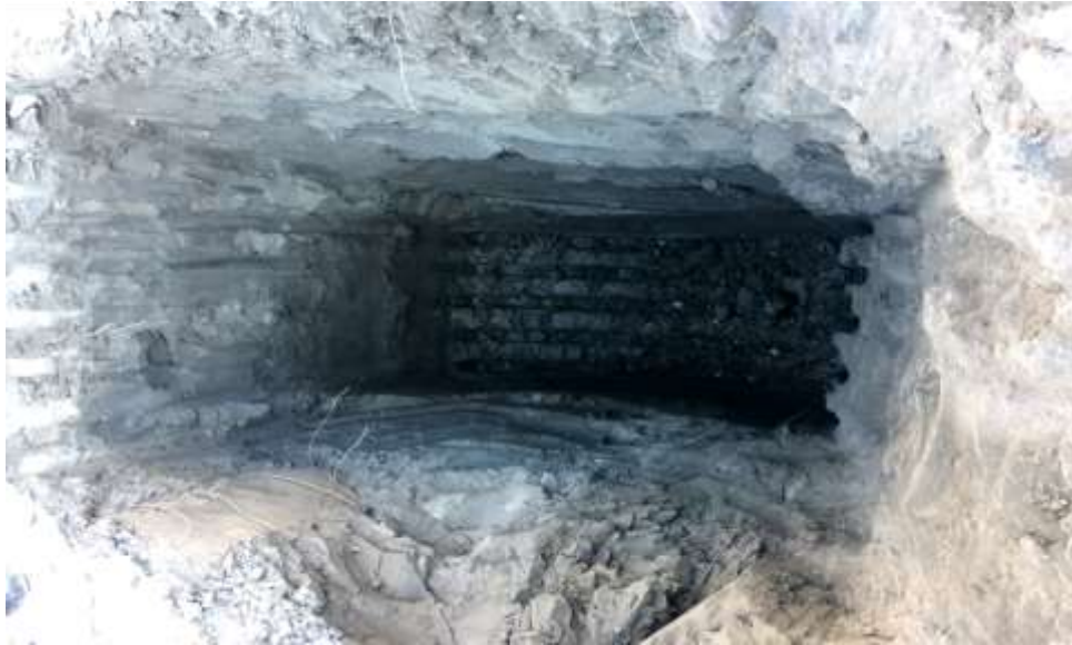
Photo 7-2 TP-3, Excavated for Clayey Silt in P/H Area.
