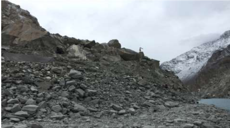
Photo 6-4 Intake Area of Sediment Flushing Channel.
