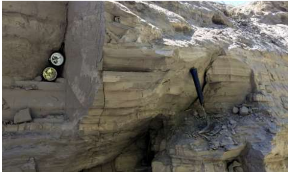
Photo 8-9 View of Vertical and Oblique Joints in Clayey Silt at Sarat Village.
